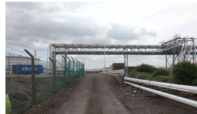
East Side Pipe Bridge
