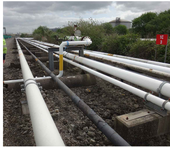
Linkline Corridor East Facing View
