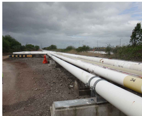
South Side Linkline Corridor West Facing View
