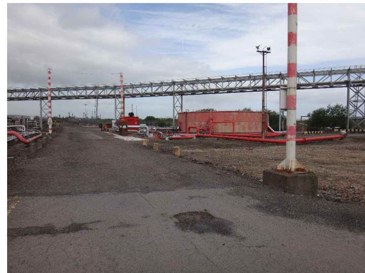
Access Road to Pipe Bridge
