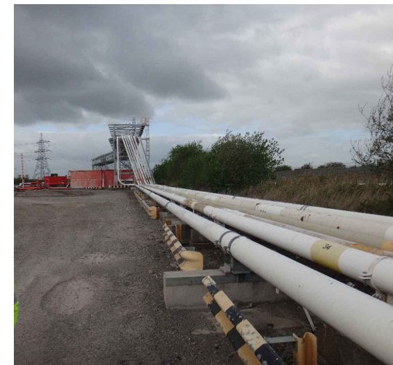
South Side Linkline Corridor West Facing View
