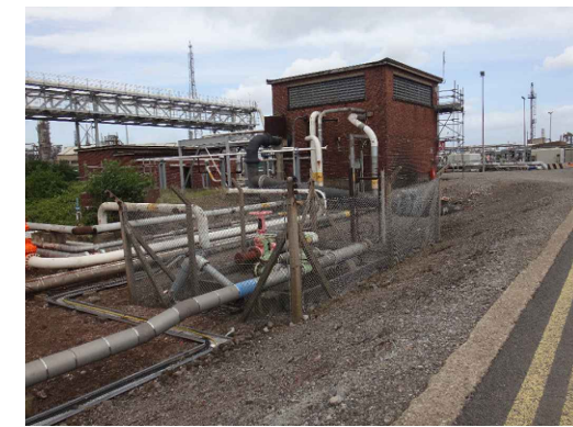
Tunnel Head House
